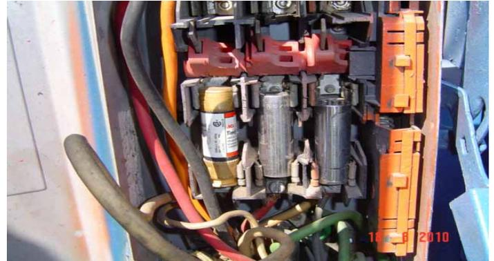
*Fuses replaced by deep well sockets. A serious fire and/or shock hazard could result.*
