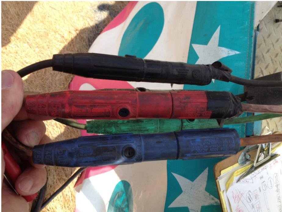
Example of “cam-lok” used with multi-conductor cable with exposed insulation. No protective jacket exists.
